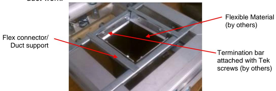
11. For each corner use the 2" wide seal material to completely cover the corners as shown below.
